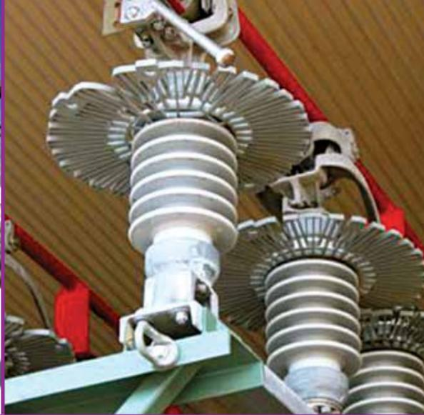
Silicone sheets and tape applied to bus while pre-molded cover designed for bushings.
