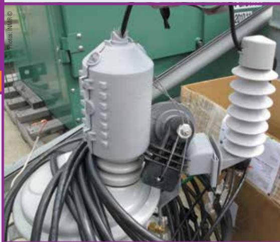
Transformer and arrester equipped with protective covers in place at time of shipment to customer.
