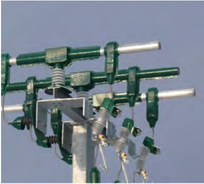
AltaLink 25kV AMI – Underground Termination
