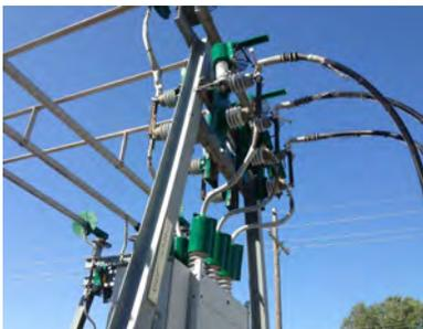
In addition to the precise-fit solution applied to existing substation equipment, Greenjacket Inc's design team worked to develop barriers for their 12kV gang-operated disconnects. The barriers are mounted to the support structure between each phase of the disconnects without affecting their operation. With the barriers in place, phase-to-phase contacts by birds and animals are prevented. Westar is considering adding the new product as a standard mitigation measure going forward.
