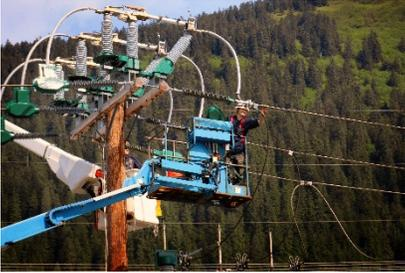
The Lemon Creek site has several generation tie transformers, distribution transformers, voltage regulators, disconnect switches, buss, jumpers, lightning arrestors, PTs, vertical orientated transmission switches, and steel poles that have unique configurations. Only the made-to-order Greenjacket product could properly protect these unique configurations.
